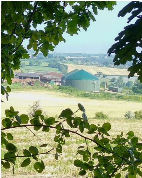
Clayton Hall Farm's Biogas Site
